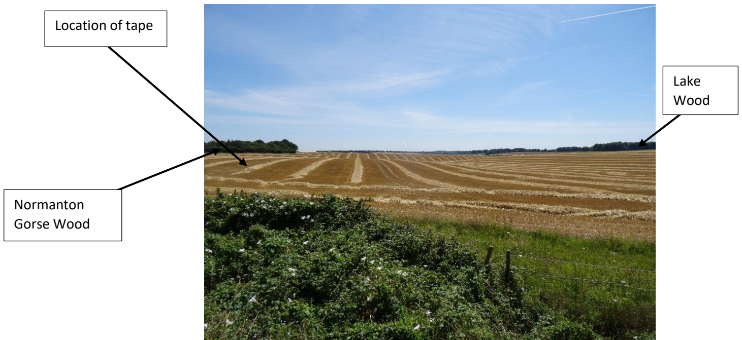
Fig 3. Photo taken from A303 verge in location of Western Portal
